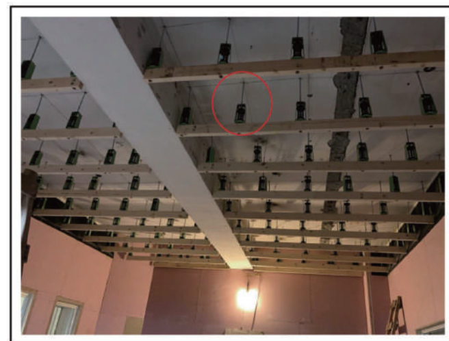
YS Spring Hangers for soundproof a ceiling
